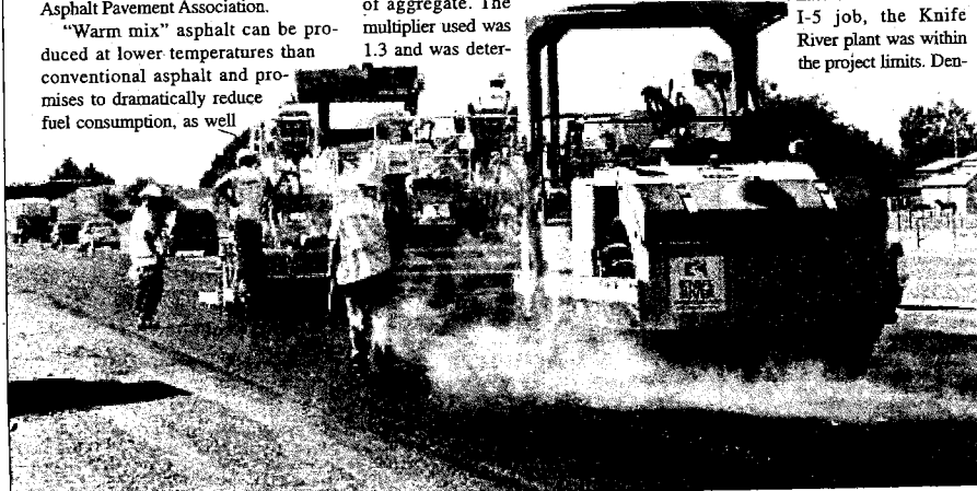
A photo of the paving operation supplied by Caltrans shows steam rising off the newly resurfaced roadway, rather than smoke.
