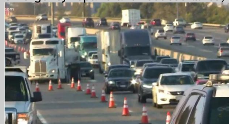
The pothole on I-5 near Sacramento disabled more than 20 vehicles and caused a massive morning commute traffic jam that made the local TV news, including this footage from KXTV Ch. 10.
