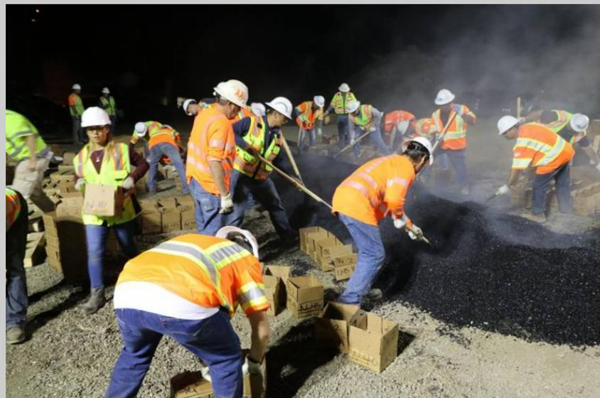
*Samplers plunge into a windrow of RHMA-G at the Knife River plant in Marysville.*
