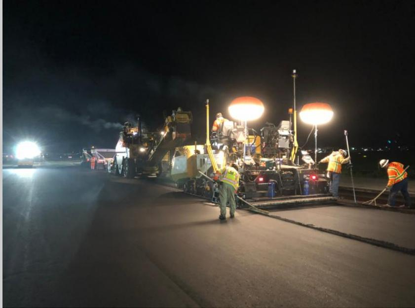
*A night paving operation achieving a smooth pavement surface, which research shows will last longer, reduce wear-and-tear on vehicles and improve fuel economy while reducing emissions.*
