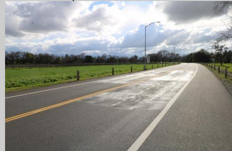
*Grinding of asphalt pavement to achieve smoothness on the campus of U.C. Davis.*
